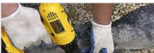
When laying out multiple pieces of PAVE EDGE flexible to create a smooth curve, it helps to drive two 1 1/4" sheetrock screws through the back support into the connector pipe. This will keep the pieces tight together as the edging is
