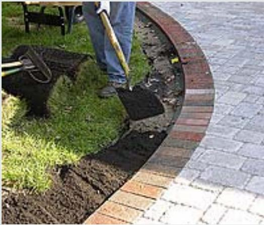
Now that the pavement is complete, it is time to cover the base extension with black dirt. Compact the dirt with your feet and fill to the top of the pavers. Then go back and cover the dirt with sod and water thoroughly for the next couple weeks to ensure the sod takes root.
