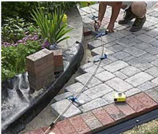
When marking body pavers along the retaining wall, we used a tool called a flexmarker. It has cleats that slide onto the joints and a flexible pole is velcroed to the cleats, 8 inches away from the wall. Then a marker is used to trace along the pole. After the body pavers have been marked and cut, the soldier course can be put in place.
