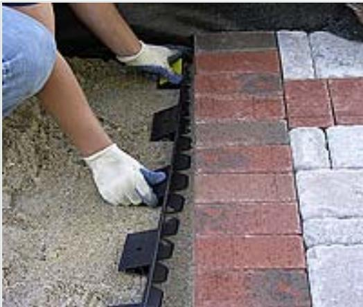
Starting at one end, place the edging flat on the base and start sliding the lip under the bedding sand until the back support is tight to the pavers. Spike the edging in with a slight toe-nail to help draw the edging tight to the pavement. When spiking PAVE EDGE flexible, regardless of the pavement application, always spike every back support (13 back supports on a 10' piece). The back supports slide, so space them out evenly before spiking.
