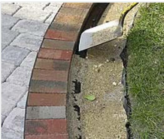
Now that all the pavers have been cut and installed, it is time to do the first compaction on top of the pavers. First place a little sand between the soldier course pavers and the edging if there are any gaps. For larger gaps, such as by the retaining wall block edges, fill the void with a little base material. Then place a little sand between gapped soldier course pavers to prevent them from twisting during the initial compaction.
