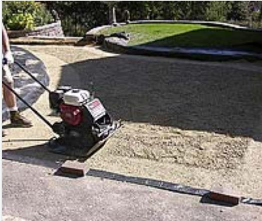
Compact the first lift by starting around the outside and work in circles toward the center. Always overlap each pass by half the plate compactor's width. Repeat this a second time, again starting on the outside. After the second compaction is complete, start compacting back and forth and diagonally.
