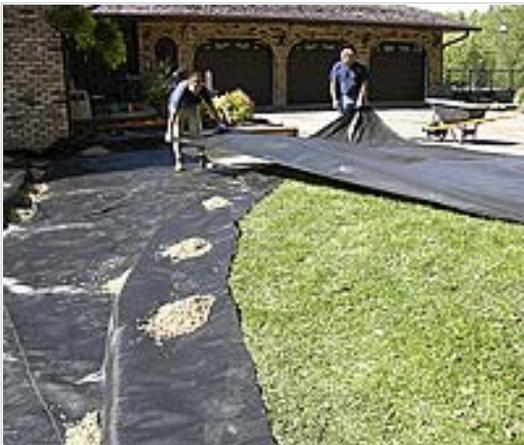
After the soil has been compacted, now is the time to install a woven geotextile fabric if required. Woven geotextile fabrics (not geogrid or weed fabric) are good insurance for clay soils and when dealing with new construction. In clay soils, it prevents the clay from pumping up into the  $\frac{3}{4}$ " minus base material and degrading the strength.
