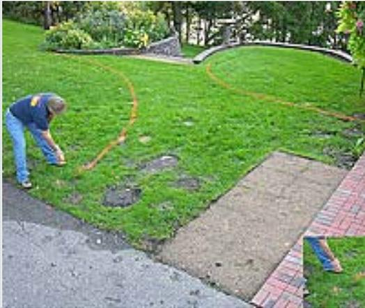
This required a total excavation of 9" from top of pavement (6" base, 3/4" of bedding sand after compaction and 2 3/8" for the paver).
