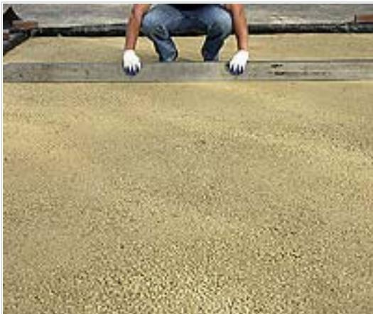
Move the pipe or board around the area checking for deviations to determine which one it is. In areas that transition slopes quickly, there are exceptions to this rule.
