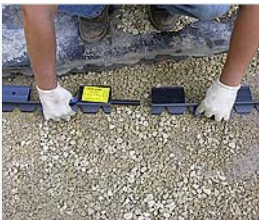
Pave edge rigid & flexible both use the same 3/4" connector pipe for attaching sections together. This connector pipe comes in long pieces and it is cut into 8" pieces and inserted into the end of the edging. It is critical that the connector pipe is used to ensure continuous strength from section to section.
