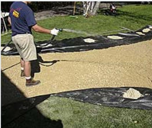
Water works as a lubricant to move the base particles together. Too little water and compaction will add air to the base and fluff it up. Too much water and the base will act like jello. The simple test for moisture content is the squeeze test. Pick up a hand full of the base material on the job site and squeeze it together. If it falls apart when you open your hand, it is too dry. If it stays clumped together, there is enough moisture. If water runs out, there is too much water.
