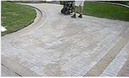
the pavement with a push broom as the compactor is run. If there is no sand over the joint, it is a wasted pass with the plate compactor. Be careful not to leave piles of sand for the plate compactor to run over. The pavers under the piles will be pushed down further into the bedding sand than the rest of the pavement.
