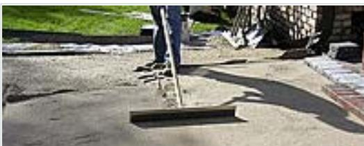
Without walking on the sand, fill the void in the sand with a shovel (only use as much sand as necessary, no more). The sand in the voids will need to be leveled with either a trowel or a sandpull. If using a trowel, touch-up the sand as the pavers are laid. When using a sandpull,
