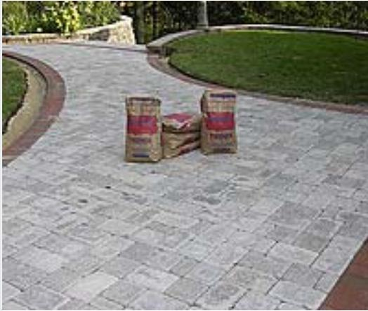
In some markets, SANDLOCK premix is available in 50 pound bags. This is proper joint sand premixed with SANDLOCK and is ready to be emptied from the bag and spread for compaction into the joints. Clean-up and activation is the same as with SANDLOCK additive.
