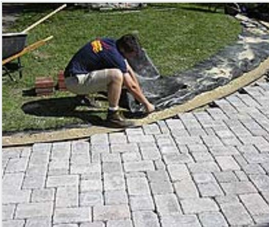
Anytime after the base installation and compaction is complete, the excess geotextile fabric can be trimmed off. Use a utility knife to cut the fabric off at the top of the base material. After trimming, if there is still fabric showing between structures, carefully use a propane torch to melt down the visible fabric.
