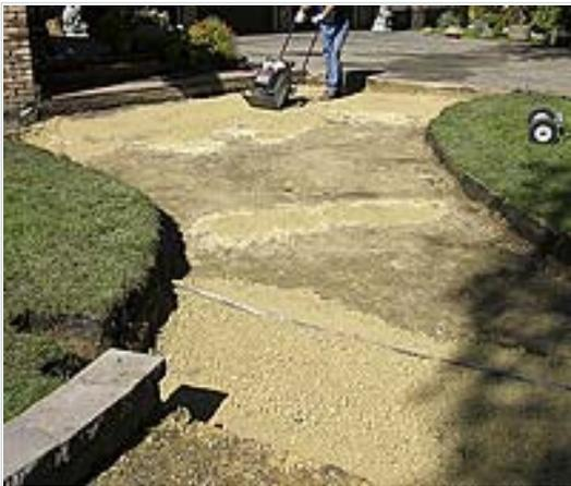
If any areas were excavated to deeply, do not put soils back in to fill the low spots. Fill these areas with base material and then compact. In order to make sure that the pavement moves uniformly during freeze thaw cycles and under loads, a consistent base thickness is required.
