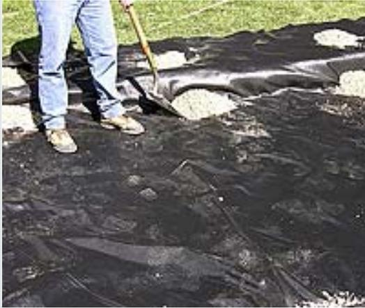
Overlap, or shingle, the layers 12" – 18" over each section. Be sure the run the layers of the fabric up the walls and out of the excavation (don't just line the bottom). By creating this "bowl" of fabric, when stretched tightly, it will provide a safety net in case the sub-soil settles. The fabric will support the weight of the base, bedding sand, pavers and the traffic on top of the pavers.
