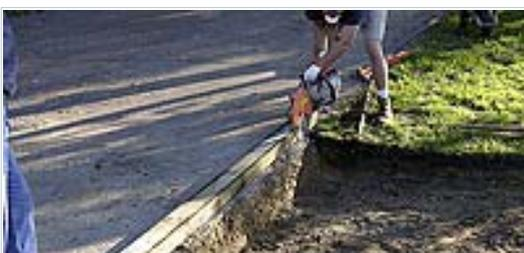
This project had one edge that was laid against an existing asphalt driveway which was not a smooth straight edge. A chalk line was snapped on the asphalt, following the edge of the existing clay patio. Since there was not much asphalt to cut off, a 4" x 4" board was used to help guide the hand-held saw along the chalk line.
