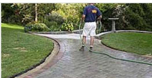
Once blown off, it is time to activate the SANDLOCK with water. Do not mist the surface; flood it with as much water as possible. Set the hose sprayer to "shower" and thoroughly wet the pavement. Once activated, the surface is safe to walk on, but it best to let it dry for at least a few hours before opening the pavement to traffic. Depending on temperature and
