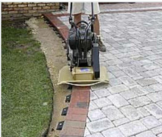
Always start compacting the pavers along the outside edging, allowing the plate to hang over the edge of the pavers. Then make circles around the pavement working toward the center. Always over lap each pass by 1/3 of the plate width. Make 3 – 4 passes around the entire pavement and the first compaction is complete.
