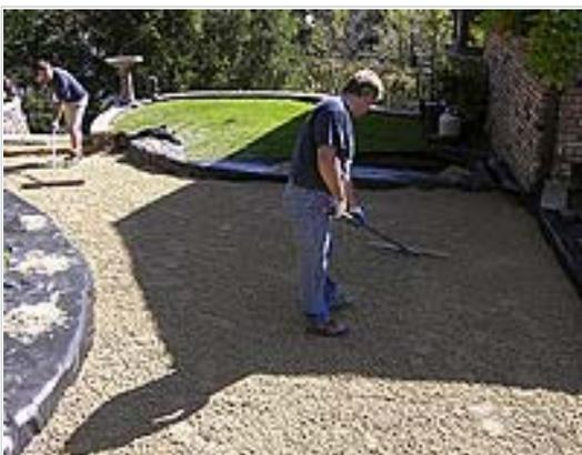
When spreading loose base material, use a baserake or another rake with a smooth, solid head. If spreading loose material with a landscape rake or other rake with teeth, the fines will have a tendency to drop out and the base will not compact properly. A rake with teeth will be needed to rough up any high spots when checking for final grade.
