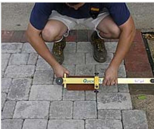
When it comes to marking and cutting pavers, there are many tools that make this easier. Since all the body pavers on a curve need to be cut, lay as many full body pavers up to the edge restraint. Then using a quickdraw, set the opening the same size as the soldier course paver. In this case, it was 8 inches for the clay paver.
