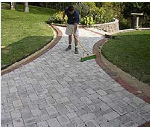
Finally, sweep of the entire pavement and start compacting. The first compaction of the pavement starts the interlock process and ensures a smooth surface. Any height deviations from paver to paver will be removed from the top of the pavement at this time (most appreciated during the winter months when the pavement needs to be shoveled). If this project only had concrete pavers, the 5000 lbs centrifugal force compactor could be run directly on top of the pavers.
