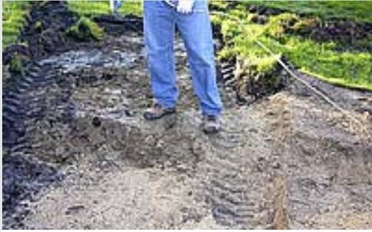
a marked utility line. For small projects such as this one, or when a skid steer can't be used, the job will need to be dug out by hand. Use a flat shovel to be able to "skim" the soil. The final excavation should be smooth and flat which is difficult to achieve with a round shovel. Keep an eye out for things like sprinkler lines and other unusual things in the ground.
