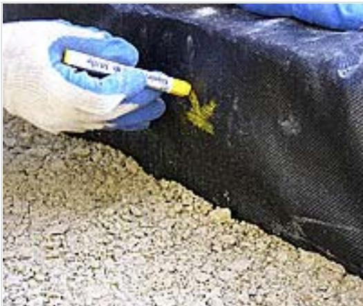
Then draw a "v" above the line, this will help to judge where the level line is without digging down to see the line. 3" is used because the 1" bedding sand will be approximately  $\frac{3}{4}$ " after compacting the pavers plus the 60 cm thickness of the pavers (2  $\frac{3}{8}$ ").
