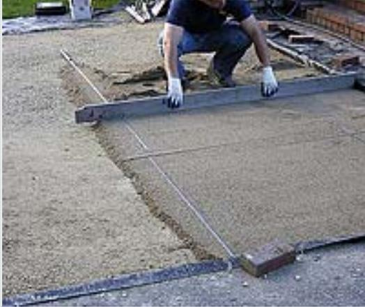
Fill the area between the pipes. The screed board is pulled across the top of the pipes to strike off the sand. In order to maintain a true straight edge on the screed board, it is best to use aluminum or magnesium screed boards or a sandpull pro.
