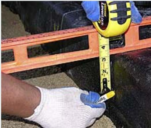
In order to help see where the final lift should stop, measure 3" down from top of final pavement. Make a mark on the side of the excavation with a line using a marker or a carpenter crayon.
