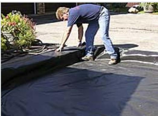
On new construction jobs, it can help prevent future settling. Only use woven geotextile fabrics between the soil and the base. Laying it under the bedding sand will not help at all and laying it between the bedding and the pavers will harm the integrity of the project. When laying the fabric in the bottom of the excavation, start at the bottom of the slope and work up.
