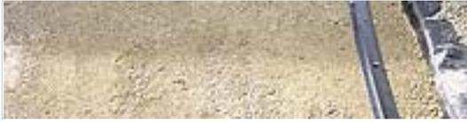
String lines are pulled across the pavement in both directions to make sure that all the bond lines are straight. Make sure the bond lines are straight before any pavers are marked and cut.
