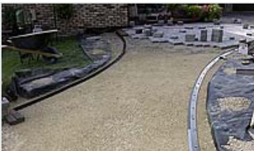
Now that the edging is set, it is time to continue laying pavers. The goal of each work day is to complete the section of pavement laid. This means that the bond lines are straight, body pavers cut, soldier course laid, edging spiked in place, pavers compacted and joints filled with joint sand. It is important to monitor progress as the work day continues.
