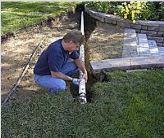
Since there may be a need to run a utility (electricity, sprinkler line, etc) to or from the house, a pvc sleeve was run under the base material. This will allow the homeowners to get under the pavement without having to tear up part of the pavement if needed. Schedule 40 pvc was used and the ends were capped with threaded ends.
