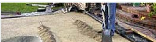
Next use a flat shovel to scrape the sand off the top of the pipes to obtain a visual idea of how much sand will be needed between the pipes for screeding.
