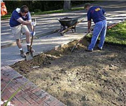
After cutting through the edge of the driveway, the asphalt and soil below was removed. Now that the soil has been excavated, it needs to be compacted. Using a compactor with a minimum of 5000 lbs centrifugal force is required. This first compaction will compact the loose material from the excavation.
