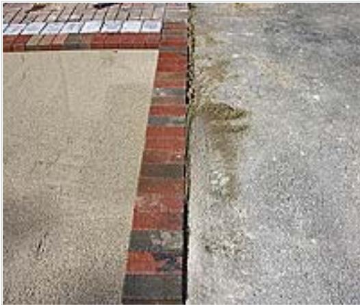
Starts by laying your "soldier" course, then follow with laying the "body" pavers. On this project, the body pavers were laid until they reached the approximate edge of pavement. When laying pavements that are curved, it is best to install the paver edge restraint first.
