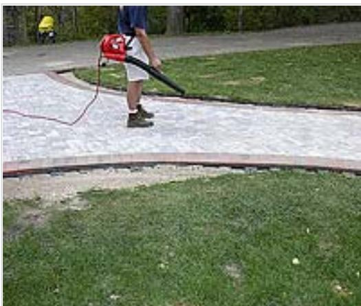
Next use a leaf blower to blow off any remaining sand and SANDLOCK from the surface. This is also the time to help contour the tops of the joints. The joint sand should be at the bottom of the chamfer (the rounded top edge of the paver), not the top of the paver.
