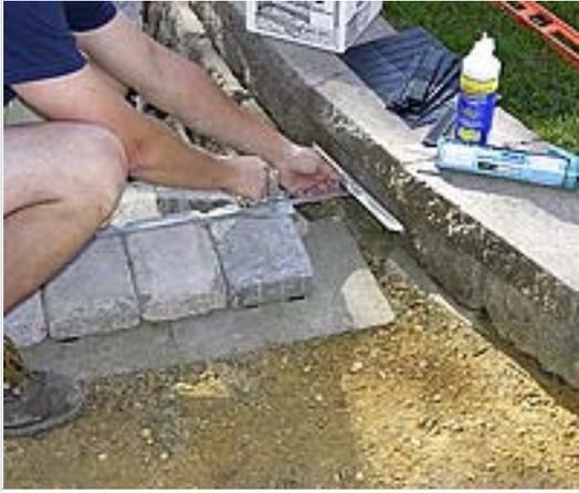
After the paver is cut, it is glued in place with a special masonry adhesive called superwet type 3. It is a foaming polyurethane adhesive that performs best when moisture is present. If the conditions are very dry, wet the surfaces to be glued before applying superwet. As with all adhesives, make sure that all dirt and debris is cleaned off the surfaces to be glued.
