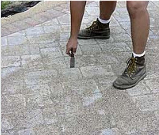
Continue sweeping and compacting until the joints are full. Stop the compactor and spot check the pavement with a 2" putty knife. Push straight down with the knife, if the sand pushes down, continue sweeping and compacting. Once the joints are full, thoroughly sweep off the entire pavement.
