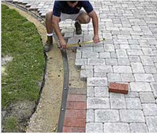
Then rest the guide on the edge restraint and mark the body pavers. Make sure to go back and put an “x” on the half of the paver being cut off.
