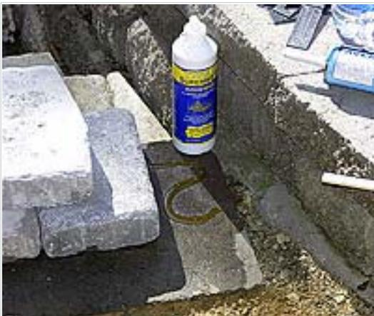
These pavers were glued directly to the existing retaining wall steps before the bedding sand was screeded. Since the retaining wall steps were sloping back to the pavement slightly, the back of the pavers needed to be shimmed so water doesn't puddle at the step. Then another moisture curing adhesive, ultrawet type 4, was used to help seal the gap between the pavers and the retaining wall block to prevent bedding sand from migrating out.
