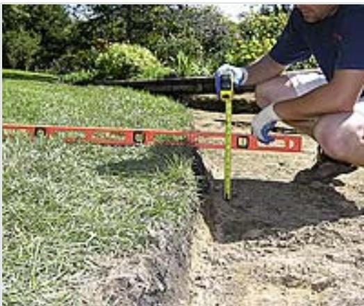
Always try to dig clean, 90 degree edges around the excavation. If the edges are not square, the final compacted base will give a false edge of excavation and the paver edge restraint may be spiked too close to the edge of the excavation.
