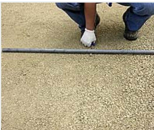
The interlocking concrete pavement institute (icpi) recommends that the base is within +/-  $\frac{3}{8}$ " over 10'. Take a carpenter's pencil and try to slide the thin side under the pipe or board. If it can not slide under, you are within proper tolerances. If the pencil fits, but there is no room to move the pencil up and down, the base is at the maximum tolerance. If there is any room for play, there is either a low spot or two high spots.
